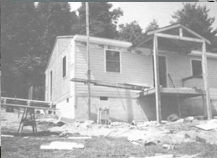
House under construction through the Buck Hill Community Improvement Project in 1995
