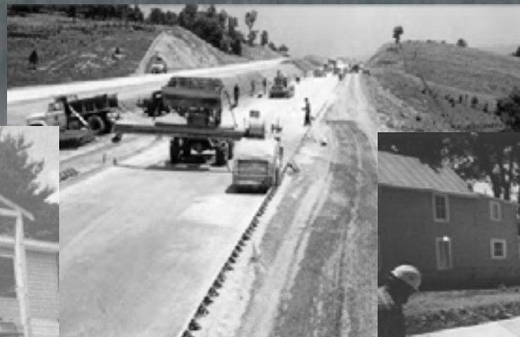
I-81 Construction in 1969
