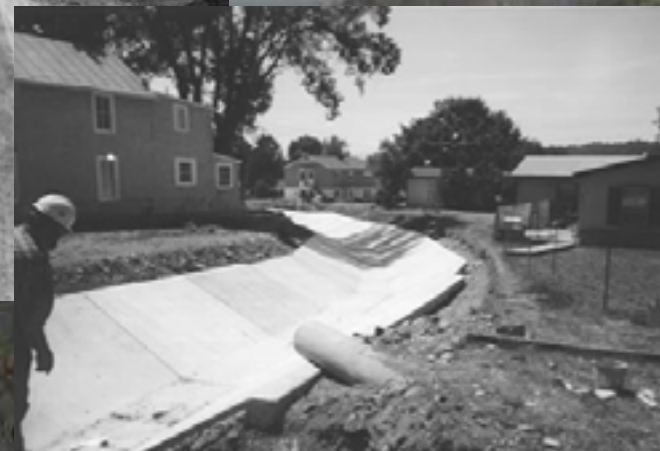
Buena Vista Interior Drainage Project in 1999
